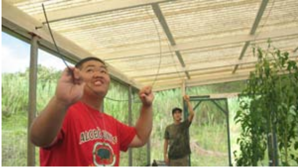
Photo: Students installing an irrigation system to hold "upside down gardens."
